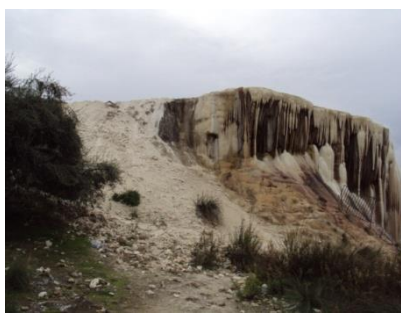
Fig .9: The collapsed
