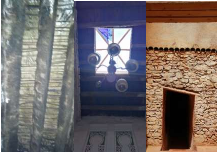
Figure 04. Architectural elements of Khizana Ezziania. (Source: Authors 2023).
