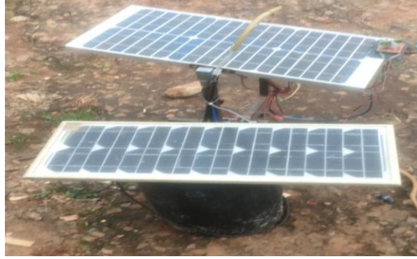
Figure 3. Fixed and hybrid tracking and cooling solar PV systems
