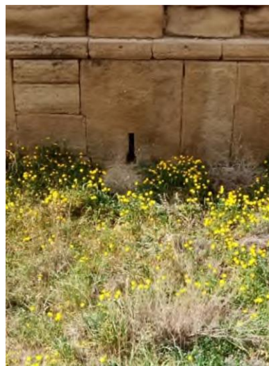
Photo n°12: Water sink of the
