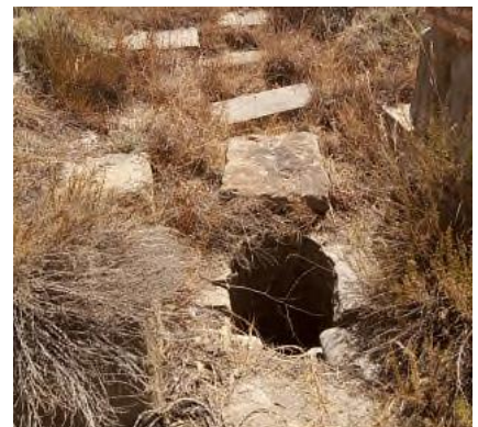
Photo n°16: water near right lateral temple
