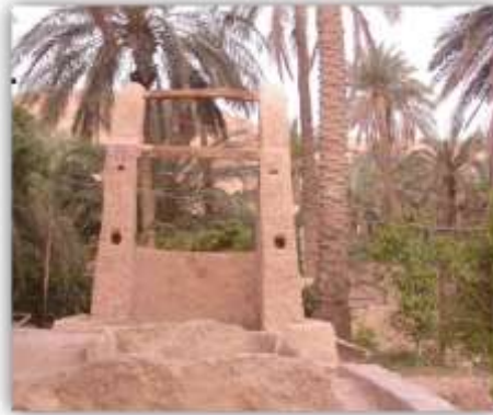
Pho.2. The superstructure of the well.
