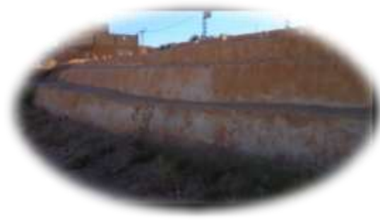
Pho.1. Remains of the Teuzouz Dam.
