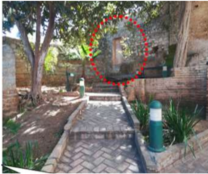
Picture 04 : A blocked door on the eastern façade of the southern garden wall
