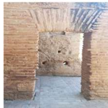
Picture : Chord Arch above Door Opening of the Rooms in the Second Wing
