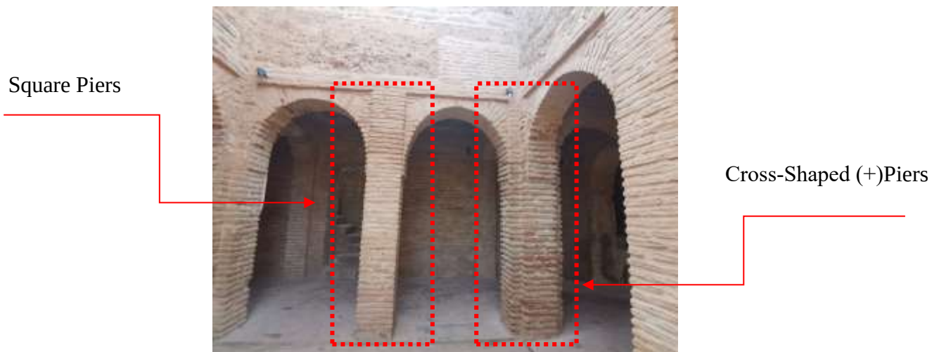
Picture15 :Cross-Shaped (+) and Square Piers in the first wing
