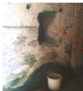
Picture :Water Outler in the Southen Wall of the Courtyard
