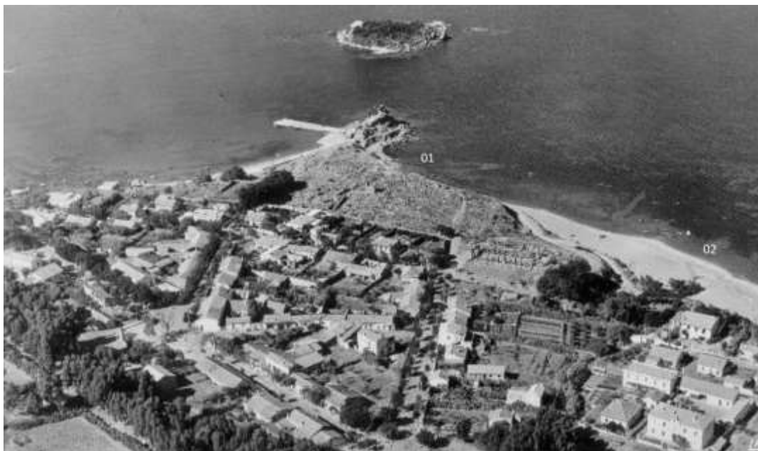
Figure 05. Oblique aerial imagery on the promontory of Tigzirt with clear submarine structures
