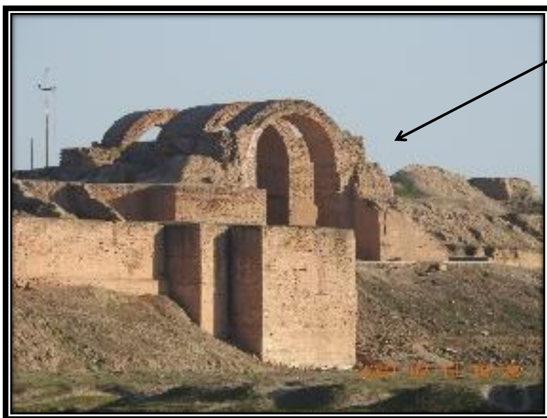
Tabira Gate after the bombing Maintenance of the first arc
