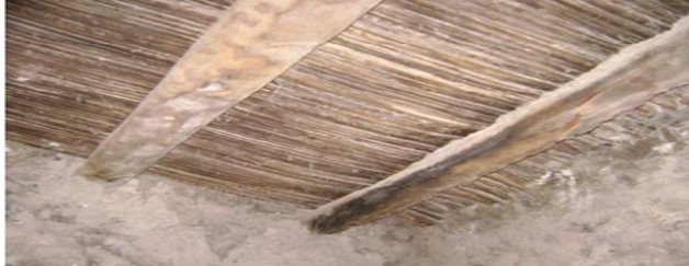
Image 05: Illustrates flat roofing using palm trunks in one of the palaces of Wadi Souf 27 .
