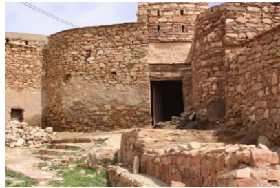
Fig.5. The Ksar's rear facade
