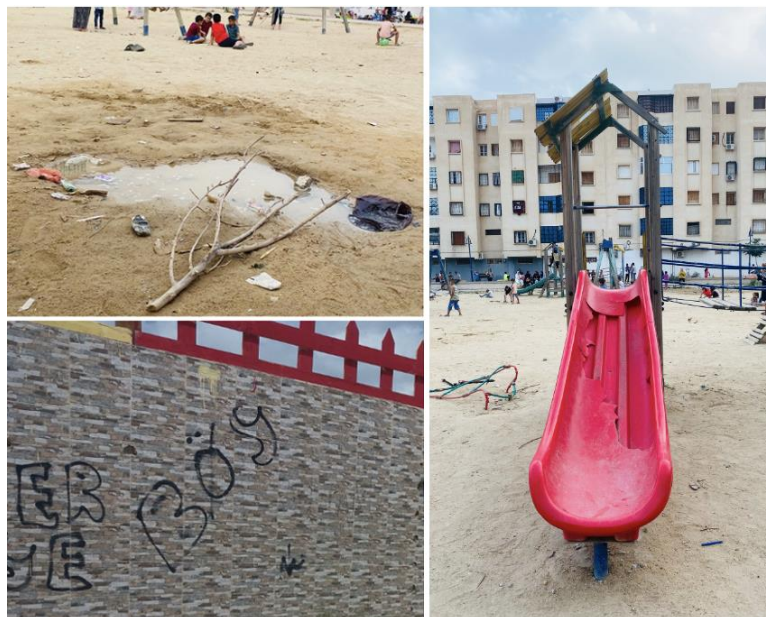
Fig.4. The deteriorated condition of the playground.
