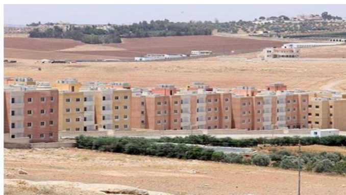
Figure (2) : the Abu Alunda housing project
