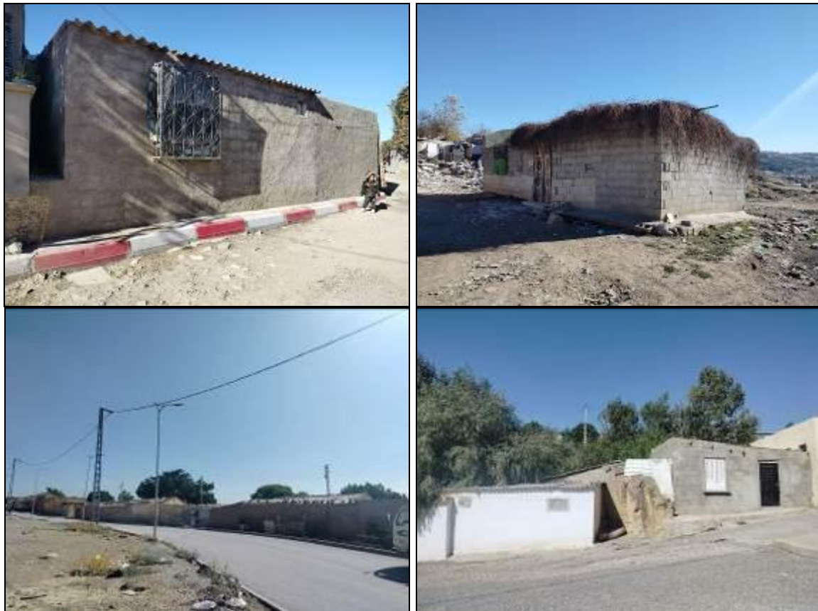
Fig.7. The deteriorated condition of buildings.
