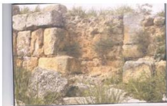
.Photo No. 5: The wall of Umm Al-Shatub Tower and its construction technique
