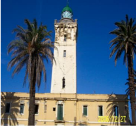
Figure 25: Ben Gouth Lighthouse
