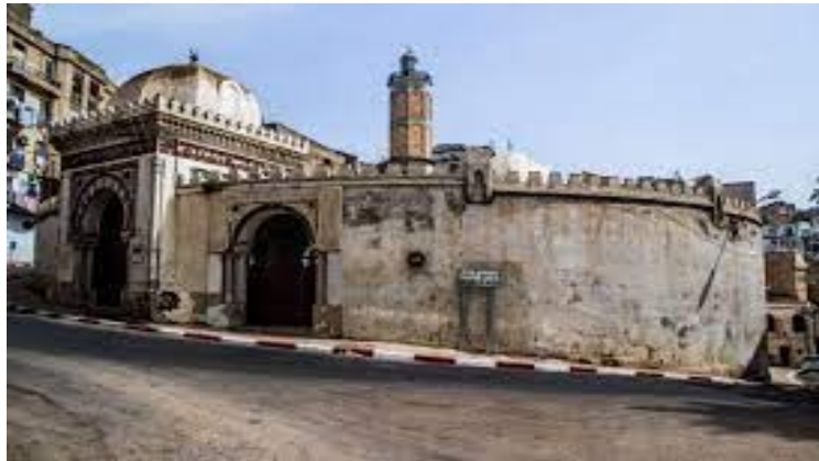
Fig.4. Hassan Pasha Mosque - Oran (West Algeria)
