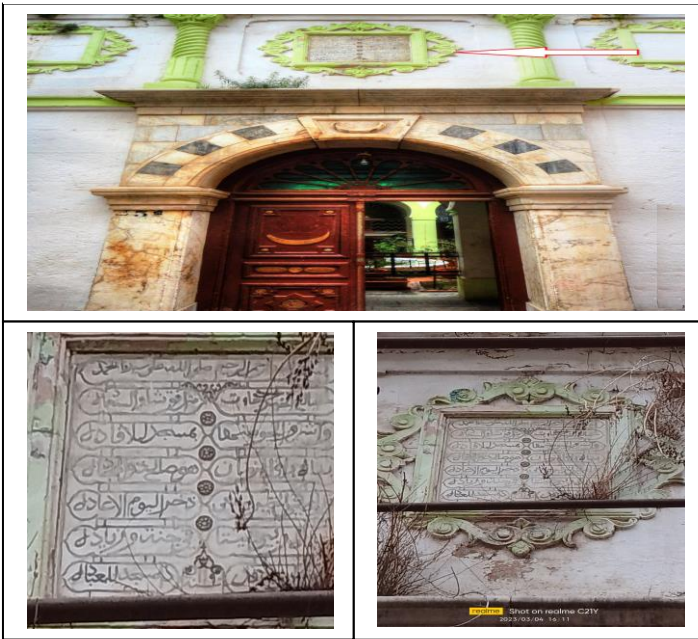
Figure No 07: The Foundational Marble Panel of the Sidi Al-Kattani Mosque above the main entrance on the southern side
