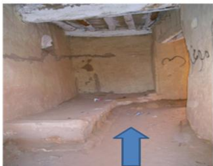
Picture N° (03): The covered shed.
