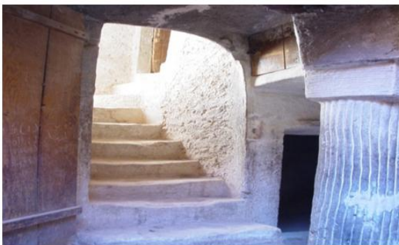
Picture N° (02): the stairs in the Mozabite house
