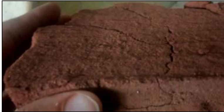
Fig. 14 – Cracking at the adobe - mortar interface.
