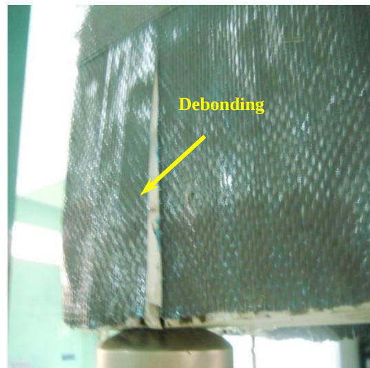
Fig. 9 – Debonding of CFRP in RS3 Specimen
