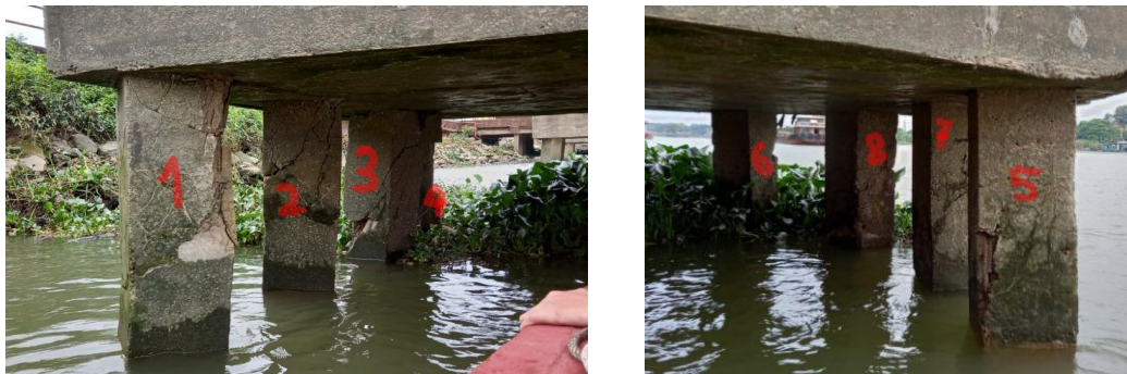
Fig. 3–Current state of dolphin piles
