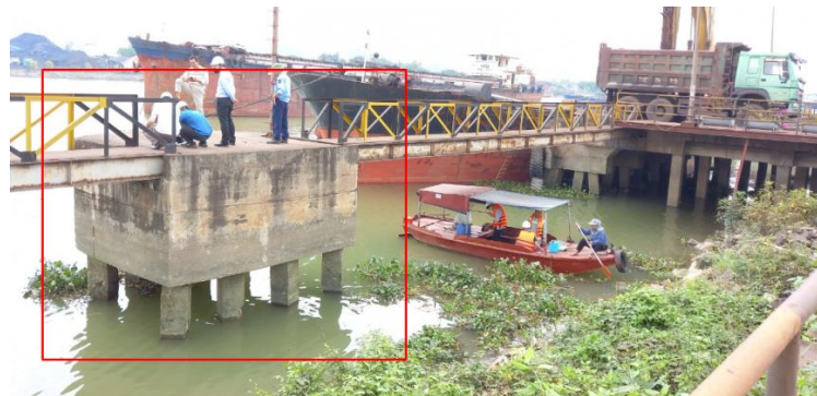
Fig. 2– Overall view of the dolphin structure
