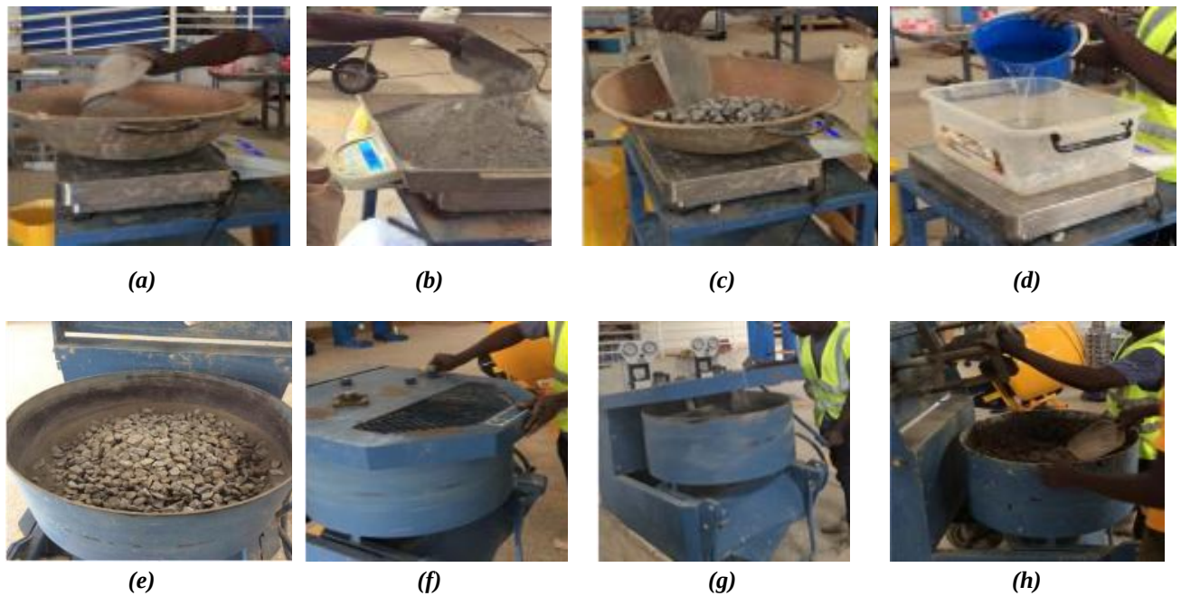
Fig. 3-- Batching and mixing material: (a) and (b) cement, (c) coarse aggregate, (d) water, (e) combination of material, (f) mixing in the process, (g) mixing of concrete, (h) concrete ready for use
