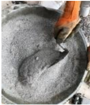
Fig. 4(c)- Before adding water, ensure that you mix the dry ingredients thoroughly.
