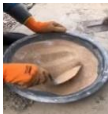
Fig. 4(b)- Before adding cement and water, mix the sand and crushed waste glass.
