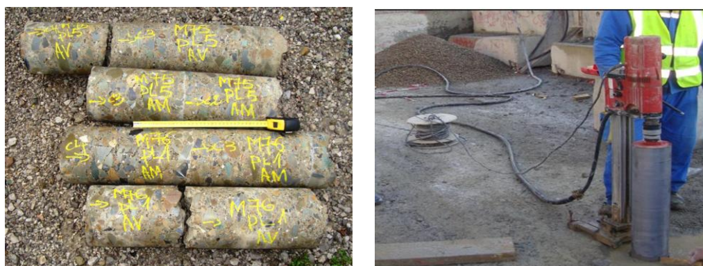
Fig. 9 – a) RCC cores taken by the laboratory on Plot 1 of Massif 76 and Plot 5 of Massif 75 with a diameter of 150 mm. b) Hilti coring machine capable of reaching a depth of 60 cm on the RCC layer.
