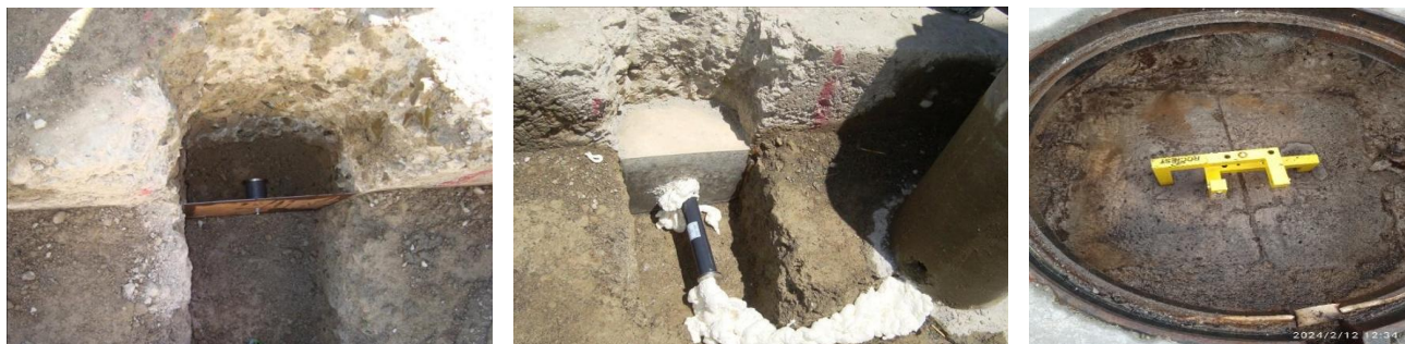
Fig. 10– Installation of the Crack Meter between Plot 4 and 5 (Before and After Sealing).
