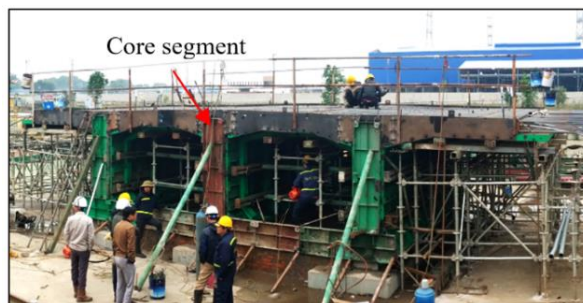
a) Core segment was cast
