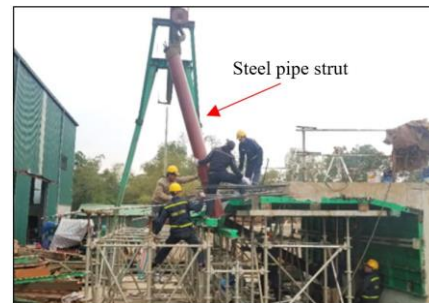
b) Steel pipe struts were erected
