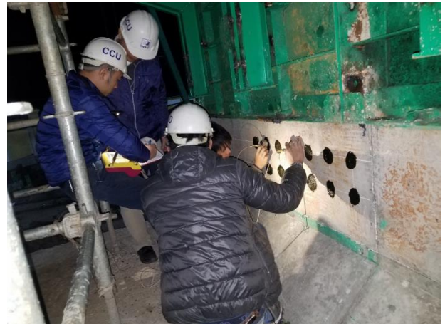
Fig. 7 - Measuring concrete strength using Rebound Hammer Test
