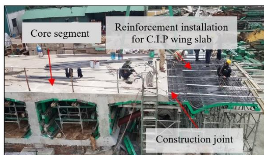
a) Reinforcement installation for the wing slab
