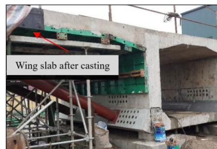
b) After the whole wing slab was cast
