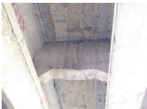
Fig. 10 – Cross beam in Kanh 7 Bridge
