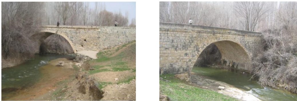
Fig. 7 – Different views of historical Sultan Suyu Bridge
