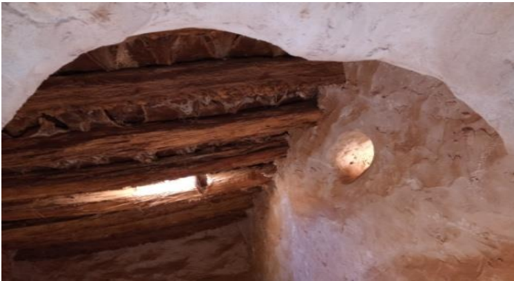
Fig.7. Lighting openings or windows
